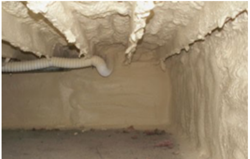
Figure 1: SFI may be applied inside crawlspaces as alternative to traditional insulation, hiding termite presence and damage.
