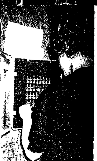
Switching On Feed Line
